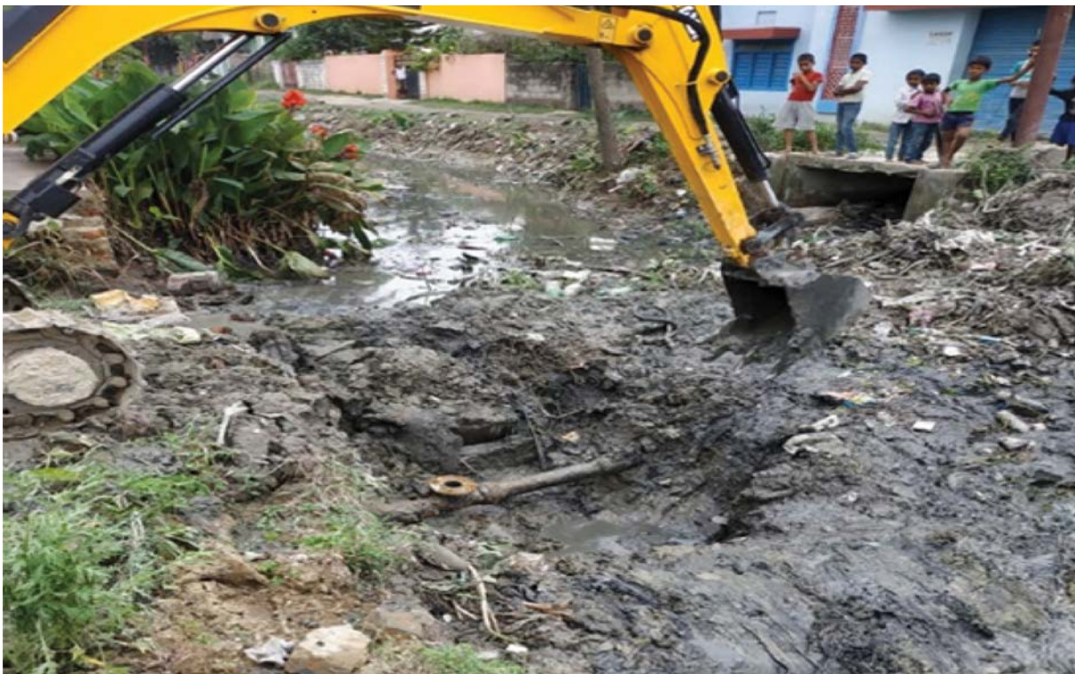
Photograph 15: Pipelaying work of Bhabardah pipeline at Lahan
