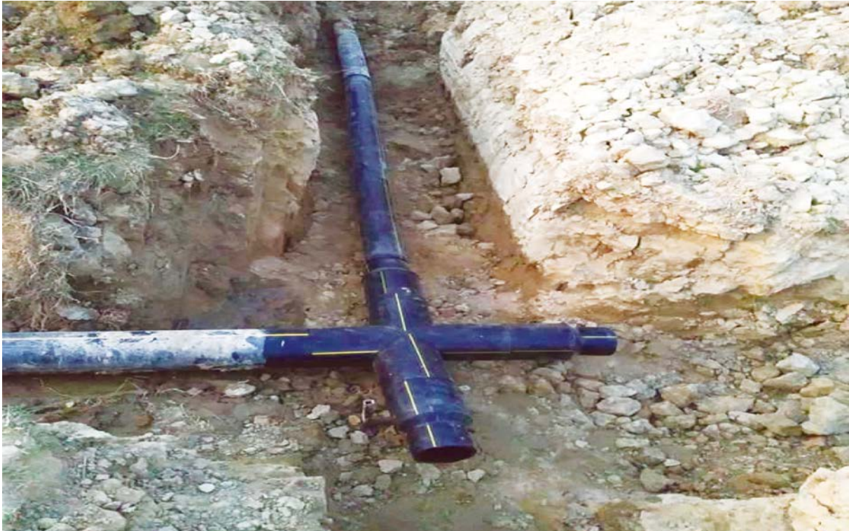
Photograph 14: Pipelaying work of Bhabardah pipeline at Lahan
