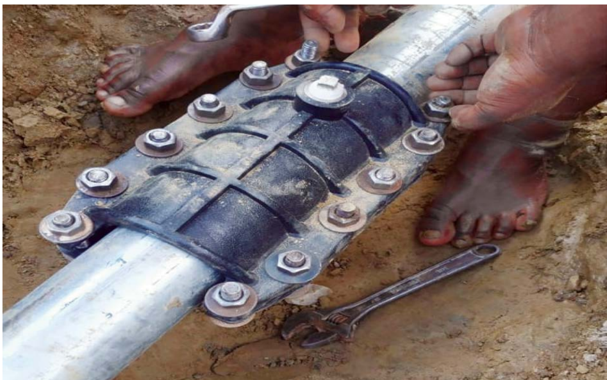
Photograph 17: Lahan Leakage
