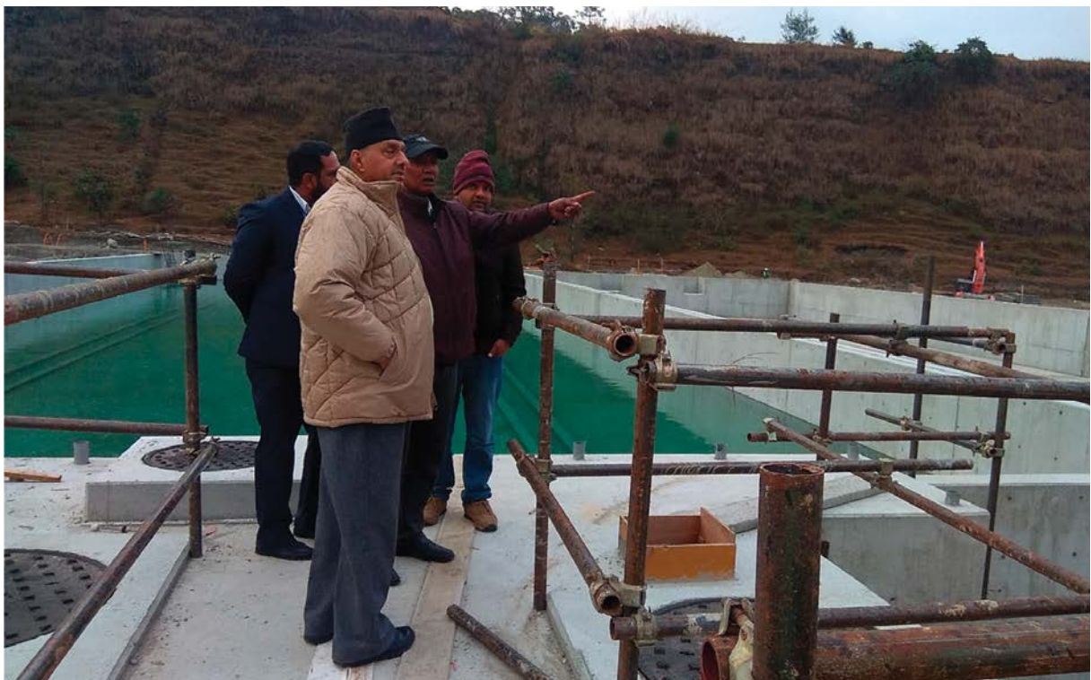
Photograph 6: Jointly Inspecting Treatment Plant, Pokhara
