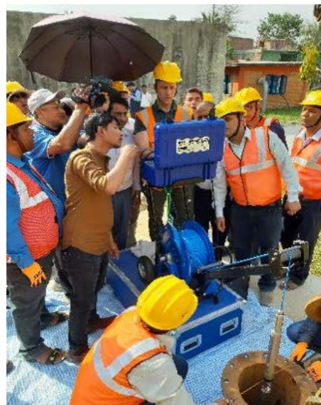
CCTV Camera Survey
