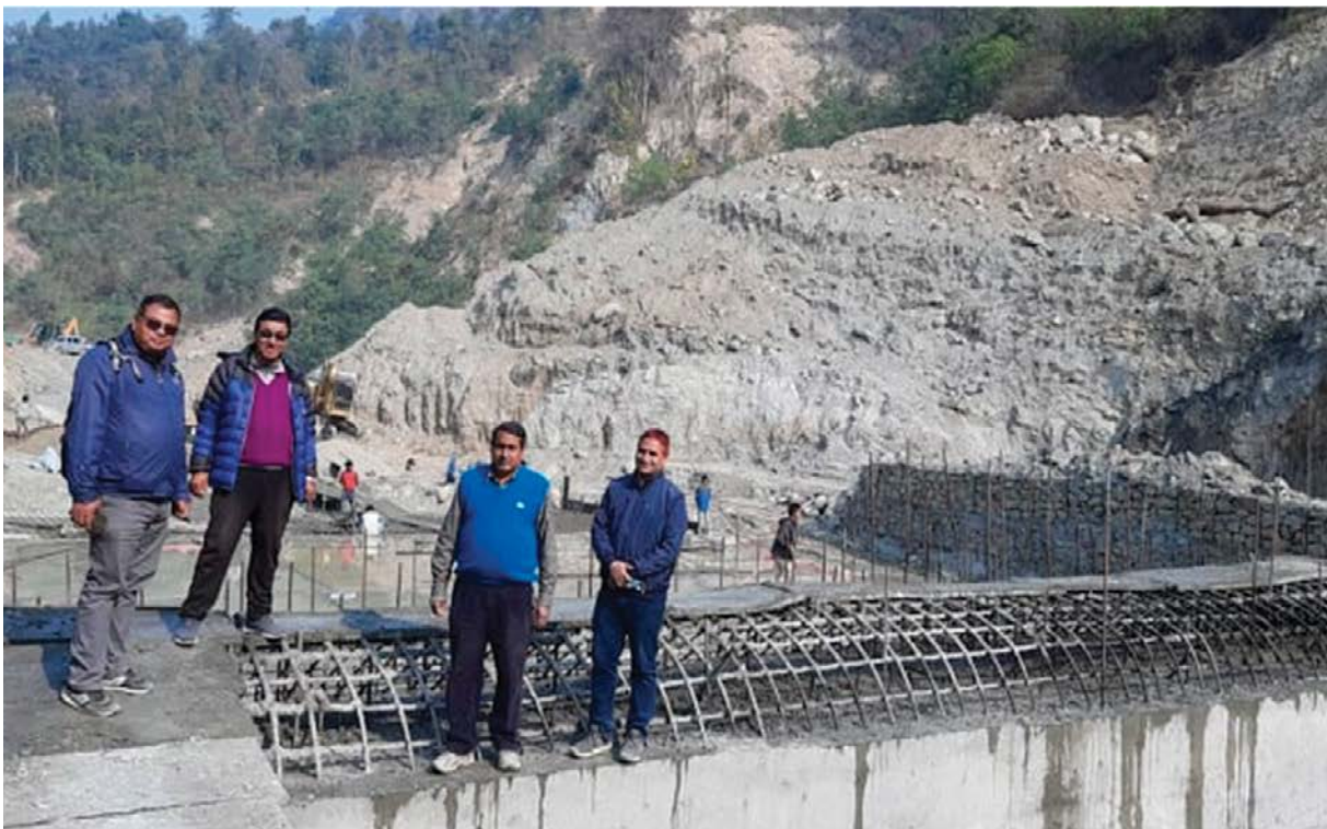
Photograph 4: Jointly inspecting construction of Dam at Jhumsa River, Palpa
