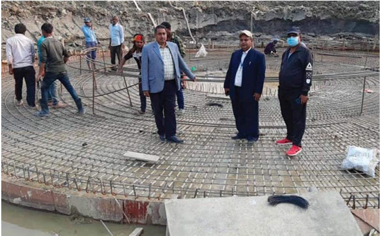
Photograph 5: Jointly inspecting construction of overhead tank at Taulihawa
