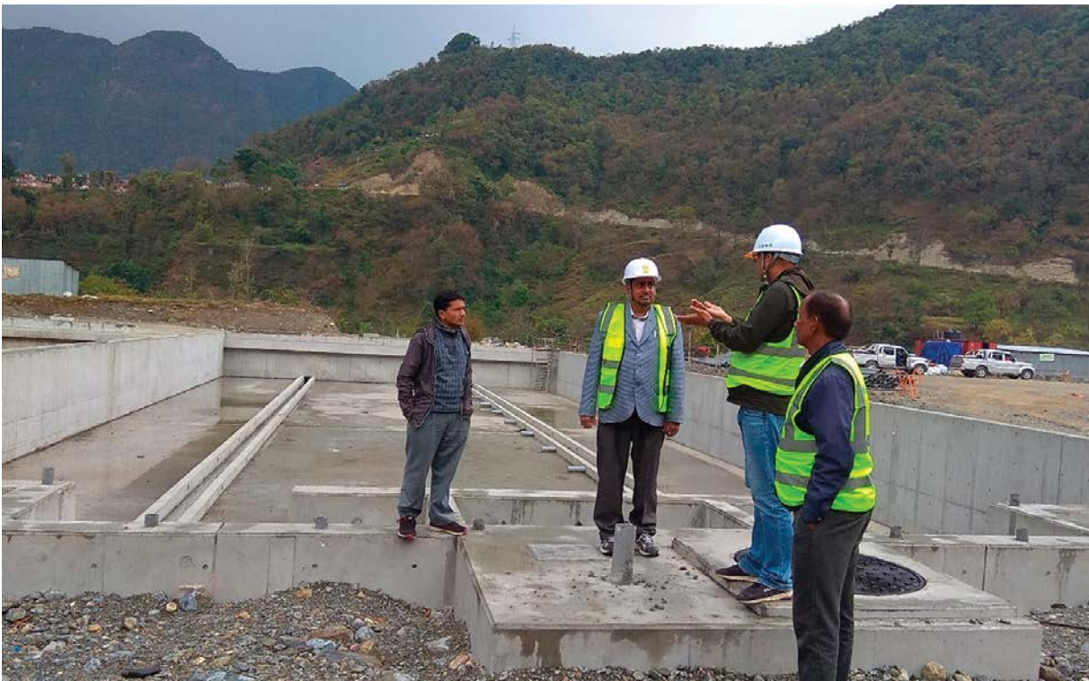
Photograph 8: Jointly Inspecting Treatment Plant (Slow Sand Filter) at Furanchaur-25, Pokhara
