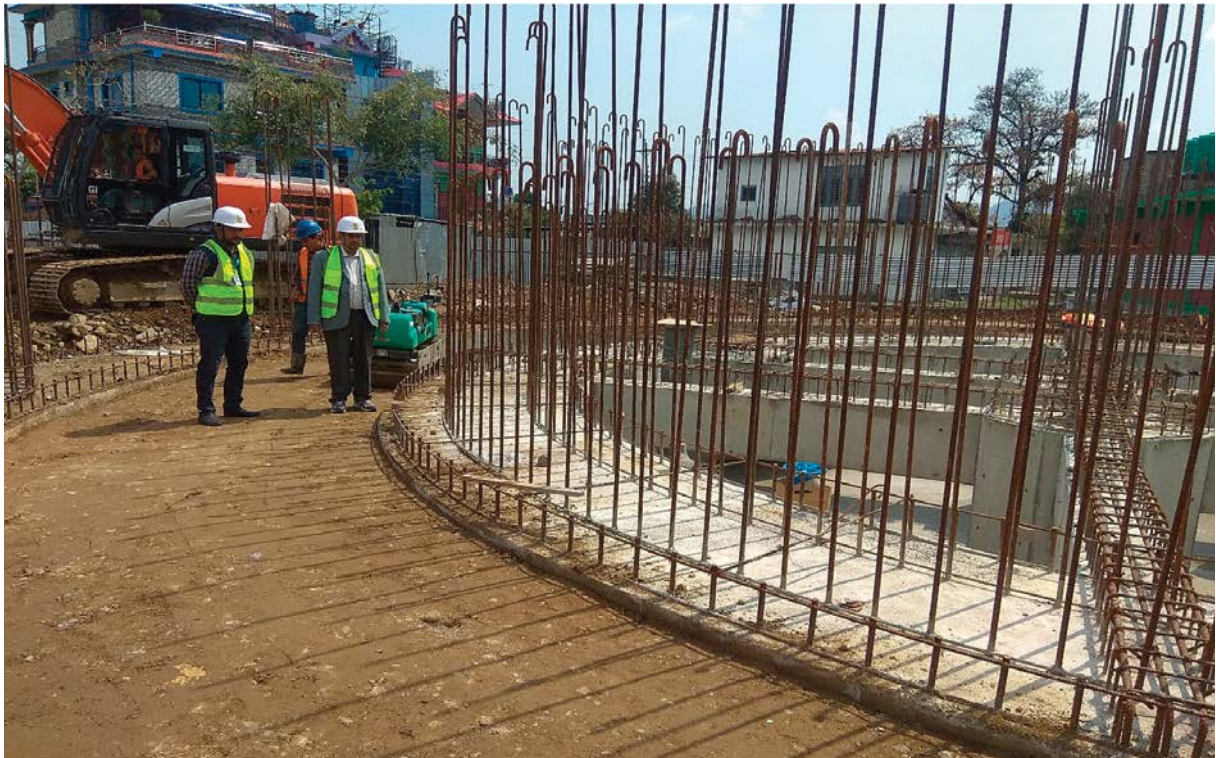
Photograph 9: Jointly Inspecting Colpatan Reservoir Foundation Work, Pokhara
